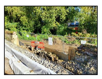
Collapsed section of Merton Priory precinct wall under repair
